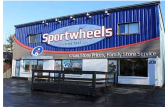
The completed façade upgrade at Sportwheels
